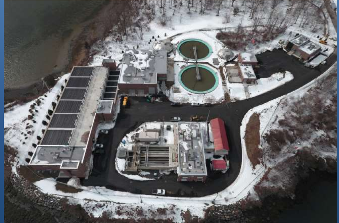
Sewer – Peirce Island Wastewater Treatment
