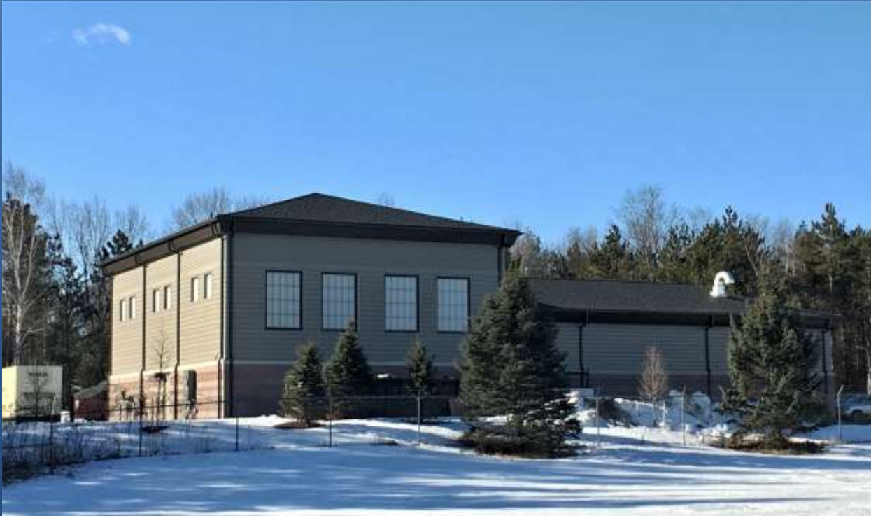
Water – Pease Water Treatment
